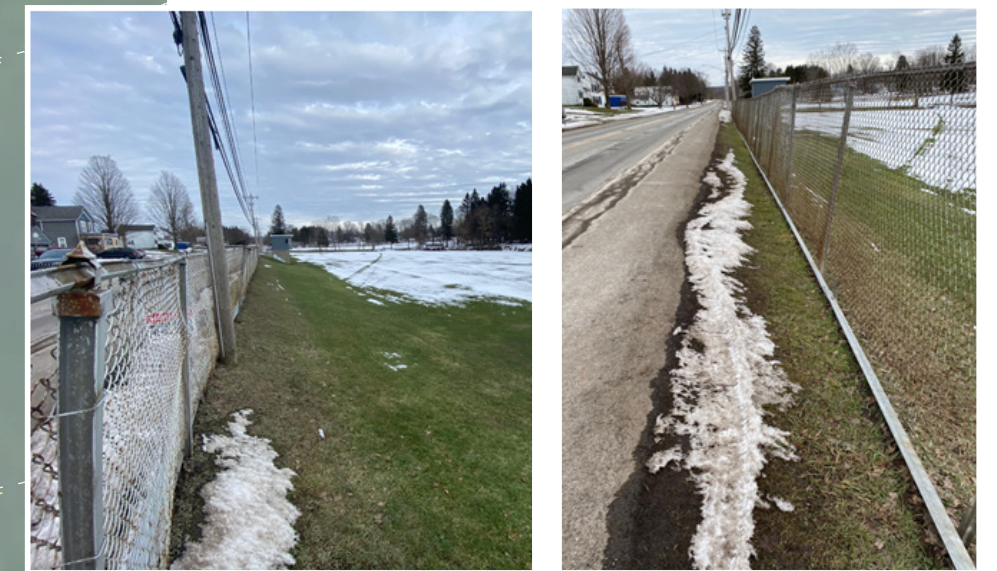
Proposed improvements will remove existing steel guiderail, chain link fence, and a portion of the paved shoulder.
